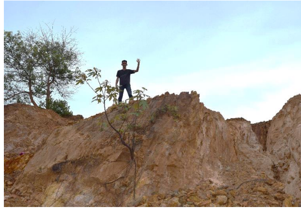
Steep cliff walls with active mining pits directly beneath make rockfall hazards and landslides almost inevitable.
