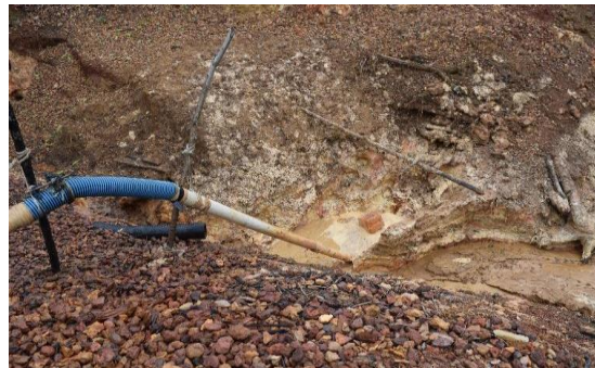
Above: Slip and fall hazards like this were observed. It would be approximately a 10-foot fall.
