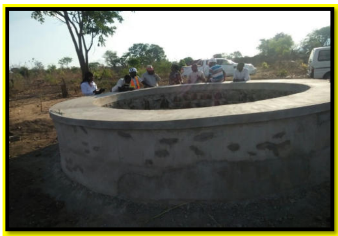
Open well without Platform and Stone Masonry Lining
