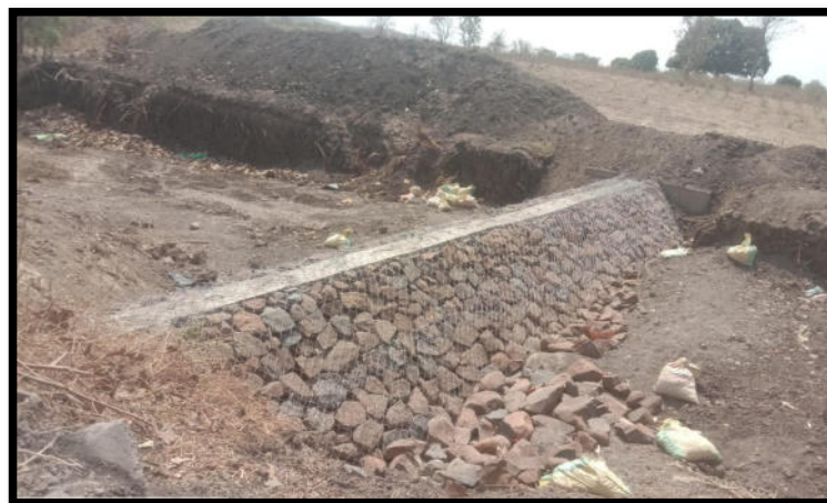
Gabion with Core Wall
