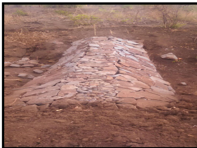
Loose Boulder Structure
