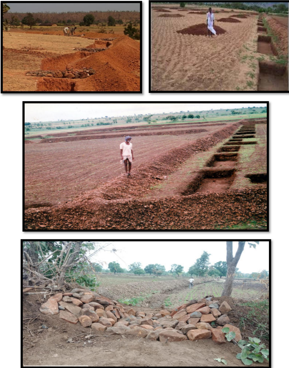
Photographs of farm bunds and loose rubble bund spillway
